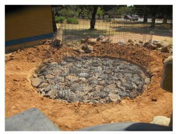
14 Attach chicken wire to the outside of the walls securing with wire ties
