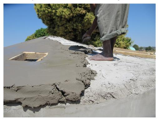
To protect the tank "chipping" takes place. A hand operated machine is filled with mortar and when turned it throws a spatter of mortar onto the surface of the tank walls creating a rough cast appearance which deters graffiti.
