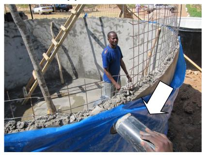
Blue plastic is wrapped round the outside of the wire walls and secured by sisal string
