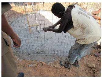
Using thicker wire at top, middle and bottom secure the structure and support the shape
