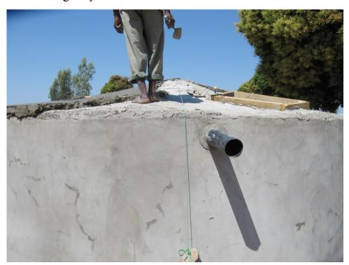
A second layer of cement is laid in sections and given a smooth finish
