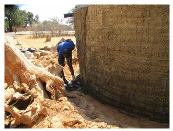
First layer of cement placed on the inside of the walls of the tank. Access is gained by a simple "A" frame ladder constructed on site
