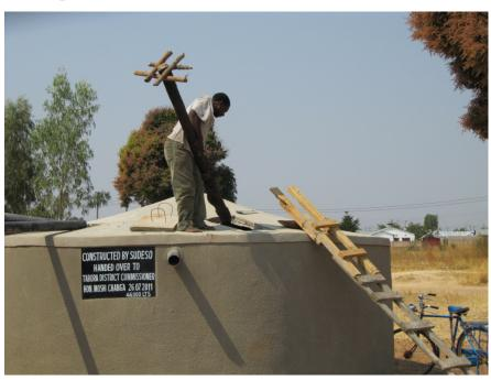
A second internal layer of concrete mixed with a waterproof agent is applied to the internal walls and dome.
