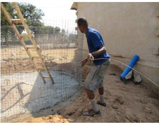
16 An overflow pipe is fixed into the wire mesh
