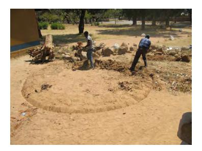
4 Place large boulders in the base of the foundations infilling with smaller stones to obtain a level surface
