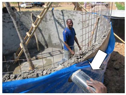
17 Blue plastic is wrapped round the outside of the wire walls and secured by sisal string
