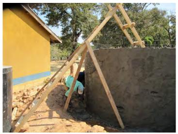
20 A second layer applied to the outside, left to set and then wrapped in blue plastic. The walls are watered for seven days so that the concrete can cure. The plastic is to delay evaporation of the water used in the curing
