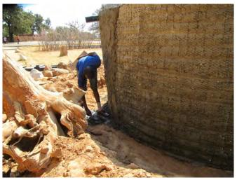
19 First layer of cement placed on the inside of the walls of the tank. Access is gained by a simple "A" frame ladder constructed on site
