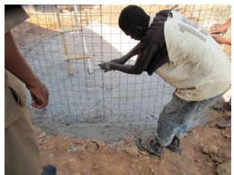
15 Using thicker wire at top, middle and bottom secure the structure and support the shape
