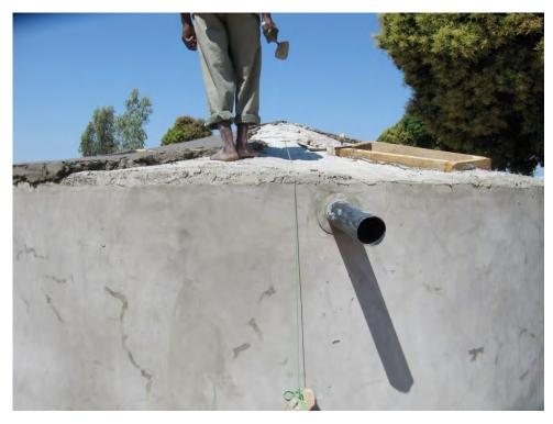
A second layer of cement is laid in sections and given a smooth finish
