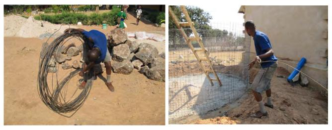
16 An overflow pipe is fixed into the wire mesh
